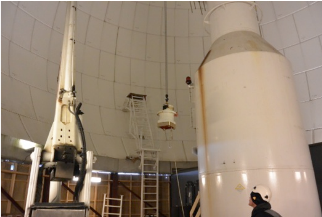
Removal of Elevation gear and motor
